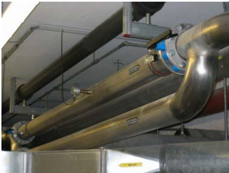
Measuring pipe with SS 20.60 at Swarovski AG (Austria) with a clever bypass solution.
